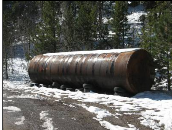
Figure 21. A 10,000 gallon cistern awaiting installation in Jefferson County
