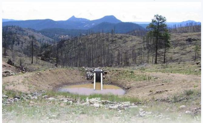
Detention ponds provide temporary volume storage from larger storm events and allow excess water to infiltrate.
