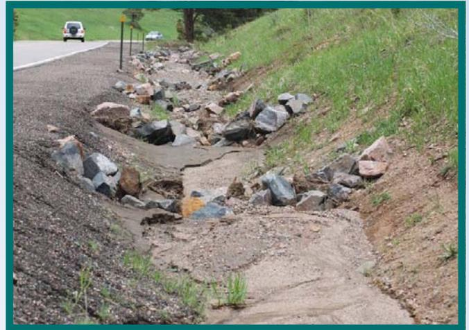
A series of rock check structures in the ditch line can provide many benefits including creating capacity and slowing runoff to promote infiltration, reducing scour, and allowing sediment to drop out in an area that is convenient to maintain.
