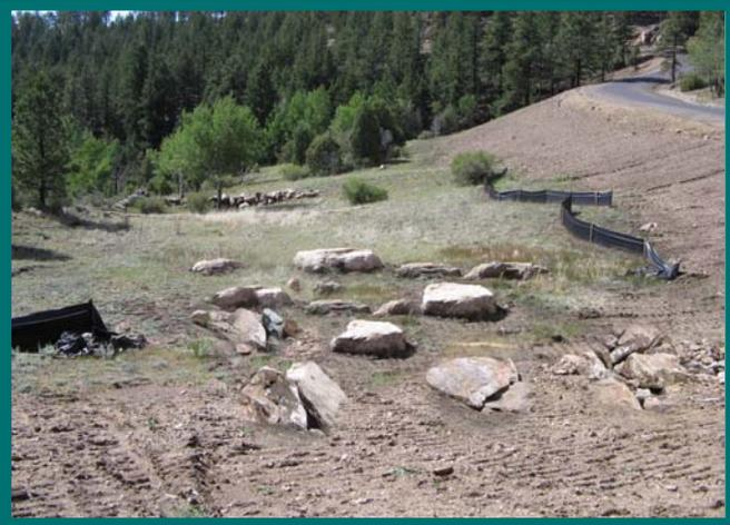
Placement of boulders and planting vegetation in the flow path help to diffuse the flow and slow it down.
