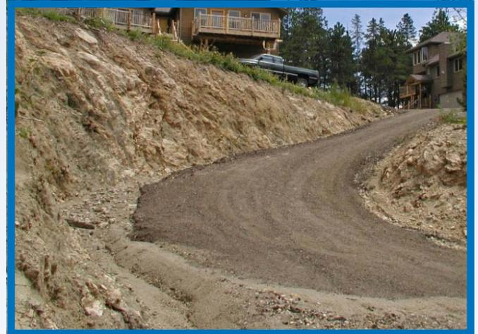
*Access roads such as the erosive driveway cut in this photo can be a source of large sediment loads.*
