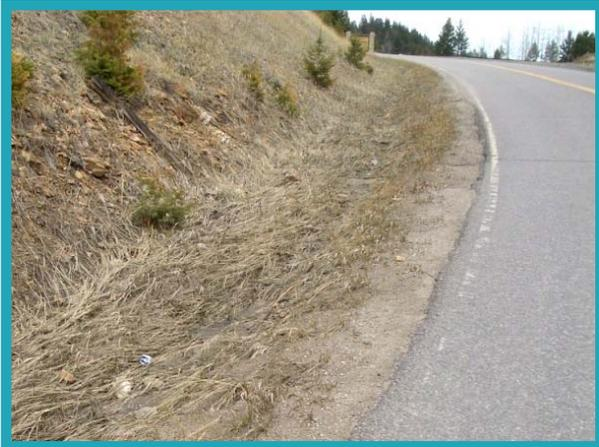
*Ditches need maintenance. When ditches fill with sediment, there is no capacity for runoff in the ditch and excess flow can cause scour downstream. ....*
